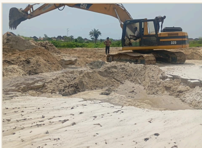
INFRASTRUCTURE — EARTHWORKS & RECLAMATION, LAGOS
